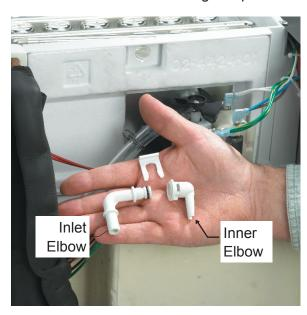
15. Pull water inlet elbow out of inner elbow.
